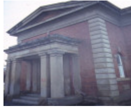
dunolly court house entrance detail aug1984
