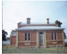
dunolly court house rear elevation aug1984
