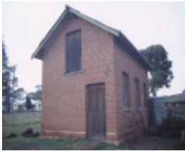
dunolly court house out building aug1984
