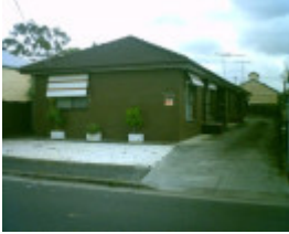
54 Albert Street Units, Geelong West
