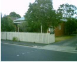
58 Albert Street Units, Geelong West
