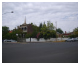
H2197 Wall associated with single story house obscured by trees
