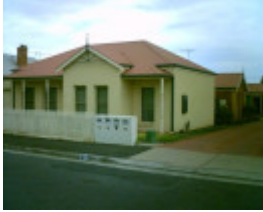
223 Hope Street, Geelong West - Units
