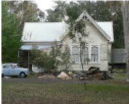
Former Corindhap State School No.1906
