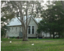
Former Corindhap State School No.1906
