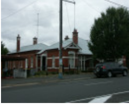
Former Bank of NSW
