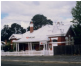
Former Bank of NSW (Westpac Bank), c.1986. Source: Linton Historical Society
