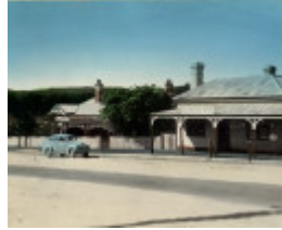
Post Office and Bank of NSW, c.1940s. Source: Linton Historical Society.
