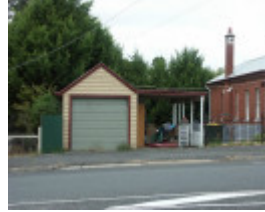
Former Bank of NSW
