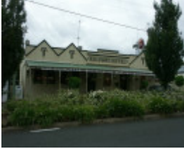
Railway Hotel (Luth's Building at Rear)
