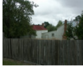
Former Blacksmith Shop
