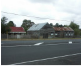
Former Blacksmith Shop
