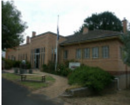
Former Shire of Grenville Offices & War Memorial
