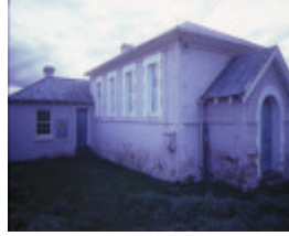
former avoca court house ballarat avoca road avoca entrance
