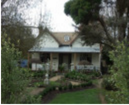
Former Post & Telegraph Office
