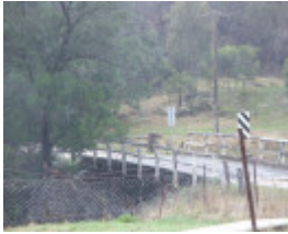
Bridge over Sutherlands Creek
