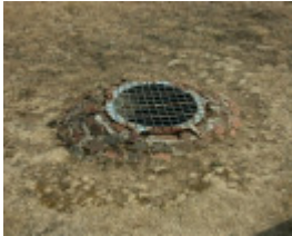
In-Ground Well, Former Hood's Bakery
