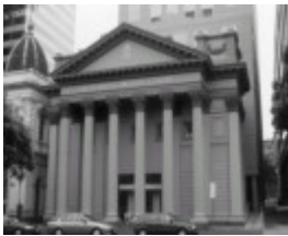
former baptist church house front elevation
