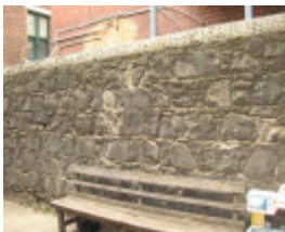
Basalt wall of coursed rubble, west boundary
