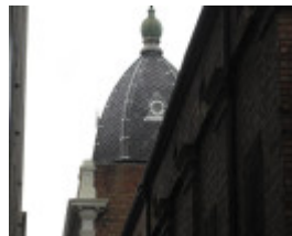
Repaired slatework to east dome Aug2014
