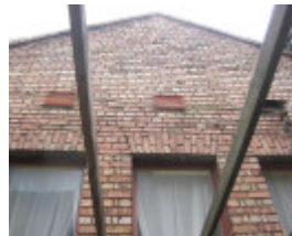
Upper west facade of school Aug2014
