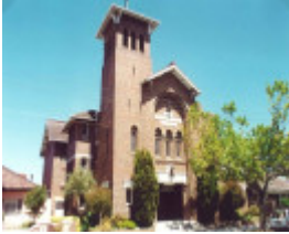
12 Ripon Grove Elsternwick, August 2000
