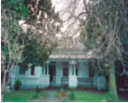
32 Booran Rd Caulfield, August 2000
