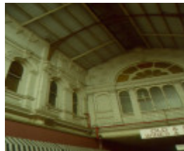
H01960 prahran arcade interior detail 2001
