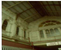
H01960 prahran arcade interior detail 2001
