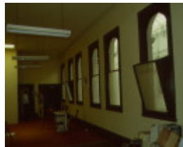
H01960 prahran arcade first floor north side 2001
