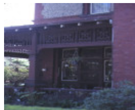
st hildas house clarendon street east melbourne verandah detail sep1981
