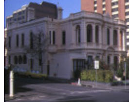
1 mosspennoch clarendon street east melb corner view
