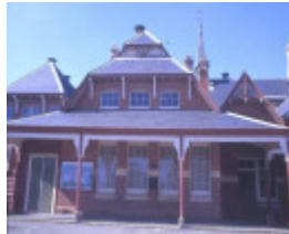
h01622 primary school no 4 barnett st avoca front of school
