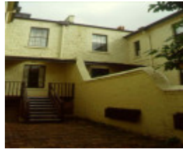
clarendon terrace rear dividing wall sw apr1999
