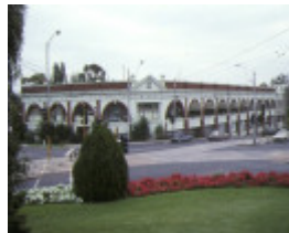
1 former hawthorn tramways trust depot front corner view
