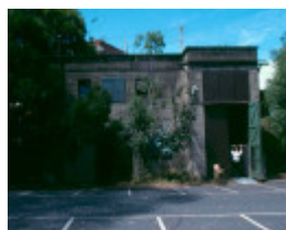
Former Hawthorn Tramway Depot Tower Wagon Shed
