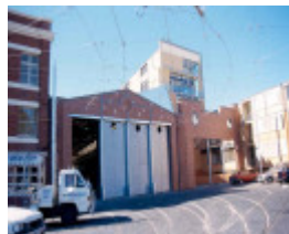
Former Hawthorn Tramway Depot During Redevelopment
