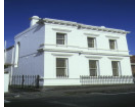
1 town house gipps street east melbourne front view
