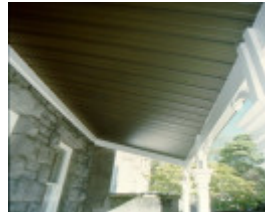
115 grey street east melbourne h58 steel decking verandah april00
