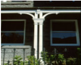
115 grey street east melbourne h58 verandah post april00
