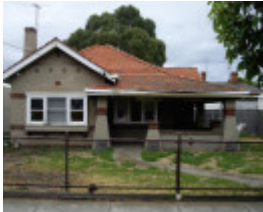
HO79 - Former Infant Welfare Centre, 95 Hamilton Street, Yarraville.JPG
