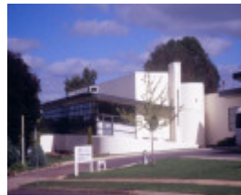
former hamilton tuberculosis chalet tyers street hamilton view from street she project 2003
