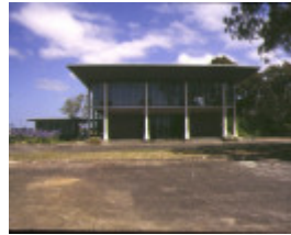
1 former bp refinery administration building the esplanade crib point front view jan1994
