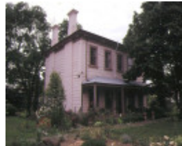
1 lyndhurst hall walhalla street coonans hill front view dec1992
