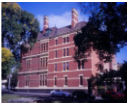
h00602 queen bess row hotham st east melbourne eastern view
