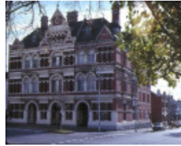
1 queen bess row hotham street east melbourne front view
