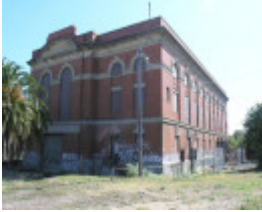
RAILWAY SUB-STATION SOHE 2008
