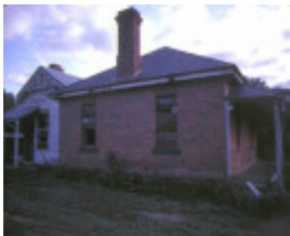
former police residence davey street avoca side view
