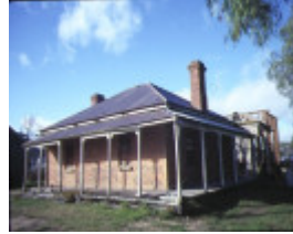
1 former police residence davey street avoca front view aug1984
