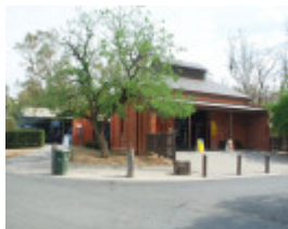
FORMER PUMPING STATION SOHE 2008
