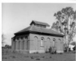
H1053 1 echuca pumping station 1964 slv
