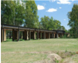
RAIL BRIDGE SOHE 2008
