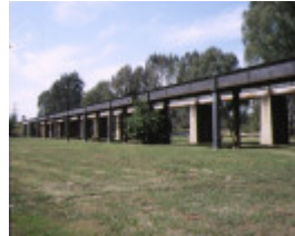
1 rail bridge benalla length of bridge apr1994
