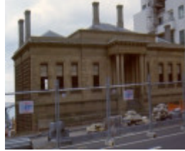
1 customs house geelong ac may00
