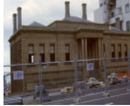
1 customs house geelong ac may00
