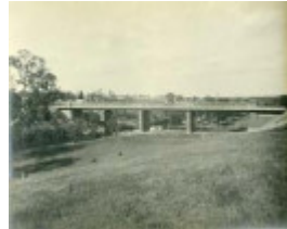
Railway bridge across the Yarra, Kew, 1891 (?) Kew.jpg
