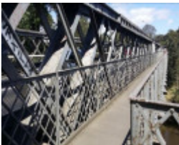
A view along the cantilevered walkway from the north looking south.jpg
