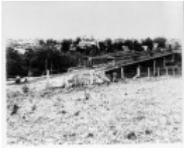
Undated photo Chandler Highway Bridge.jpg
