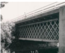
Bell Street Bridge, Coburg (1880) (Not in the VHR).jpg
