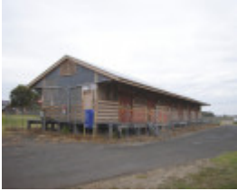
RAILWAY GOODS SHED SOHE 2008
