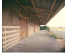
h02072 port fairy goods shed platform
