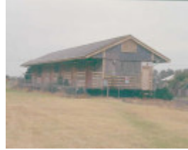
h02072 port fairy goods shed
