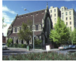
1 lutheran church external view
