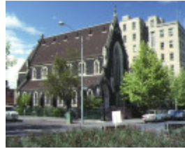
1 lutheran church external view
