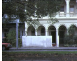
1 canterbury terrace powlett street east melbourne front view
