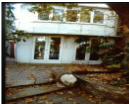
138 powlett street east melbourne h89 rear may2000
