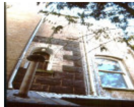
138 powlett street east melbourne h89 south elevation
