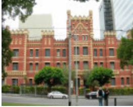
FORMER SALVATION ARMY TRAINING GARRISON SOHE 2008
