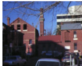
former salvation army training garrison victoria prd east melb rear view jul1982
