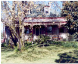
h01297 the grange belgrave street coburg front view she project 2003
