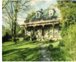
1 the grange belgrave street coburg front view sep1996
