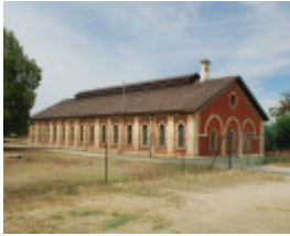
FORMER RAILWAY ENGINE SHED SOHE 2008
