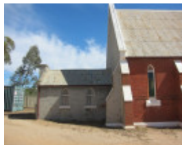
506-508 Napier Street, White Hills Uniting Church & Hall, vestry & possible early Methodist Church c1864 behind the later church
