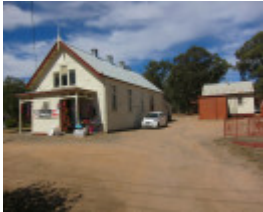
506-508 Napier Street, White Hills Uniting Church & Hall
