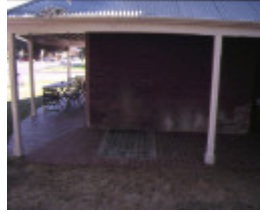
hopwood hotel echuca verandah
