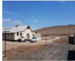
Greystones shearing shed 2019.jpg
