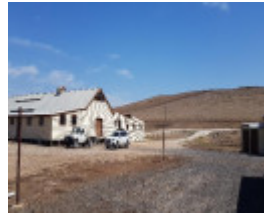
Greystones shearing shed 2019.jpg
