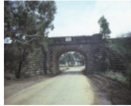
1 rail bridge & embankment geelong ballarat line elaine side view aug 84
