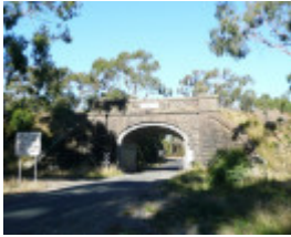
RAIL BRIDGE AND EMBANKMENT SOHE 2008
