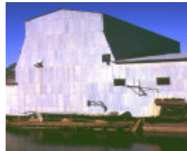
eldorado bucket dredge byawatha road eldorado rear view
