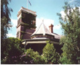
225 North Rd Caulfield, August 1994
